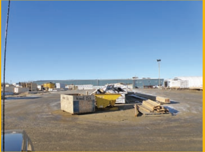
29.58 ACRES, APPROXIMATELY 25 ACRES OF WELL COMPACTED YARD SPACE
