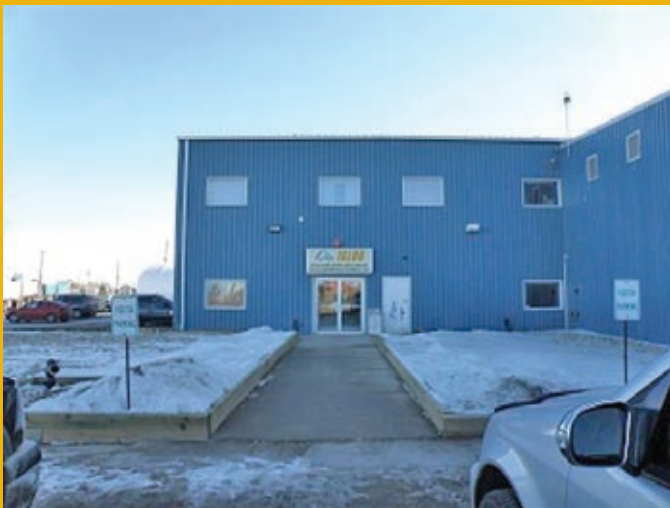
MAIN ENTRANCE OFF WINTERBURN ROAD AND CUSTOMER PARKING IN FRONT
