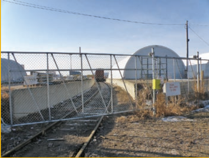
RAILSPUR C/W GATE WITH CN KEY
